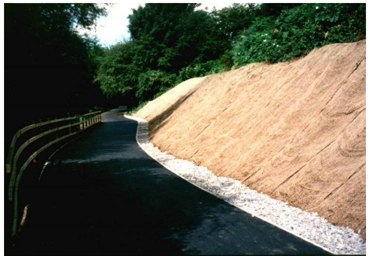
The completed cycle route with geogrids and top soil in place on the fully stabilised embankment.
