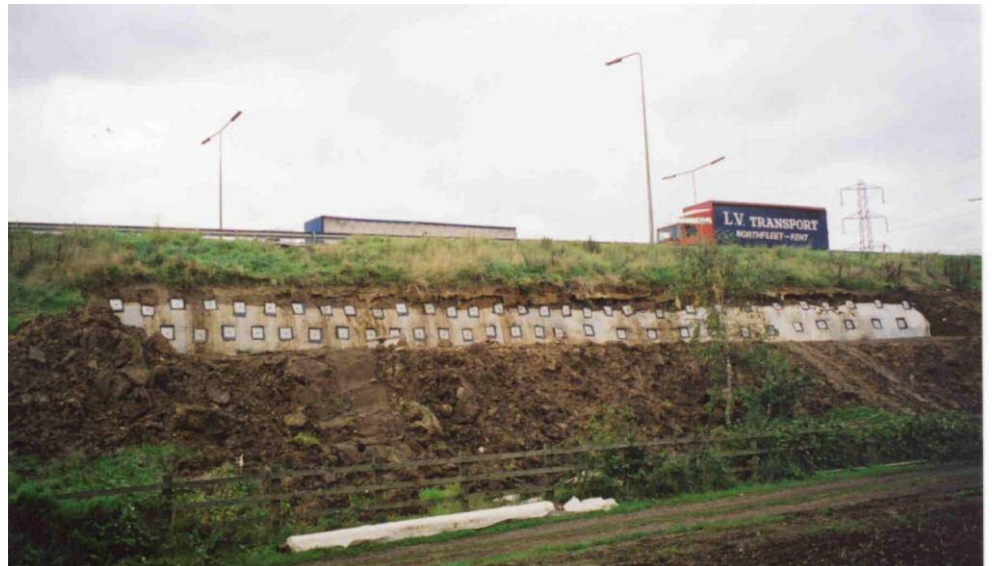
Duckbills installed in an embankment on the M25 near Junction 29, the A127 in Essex
