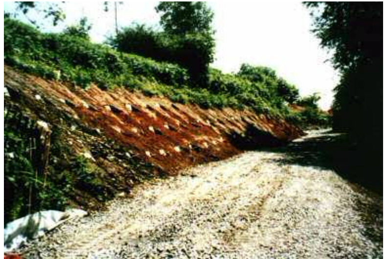
The load plates remain visible on three rows of Duckbill MR2 stainless steel anchors following installation to secure the embankment.
