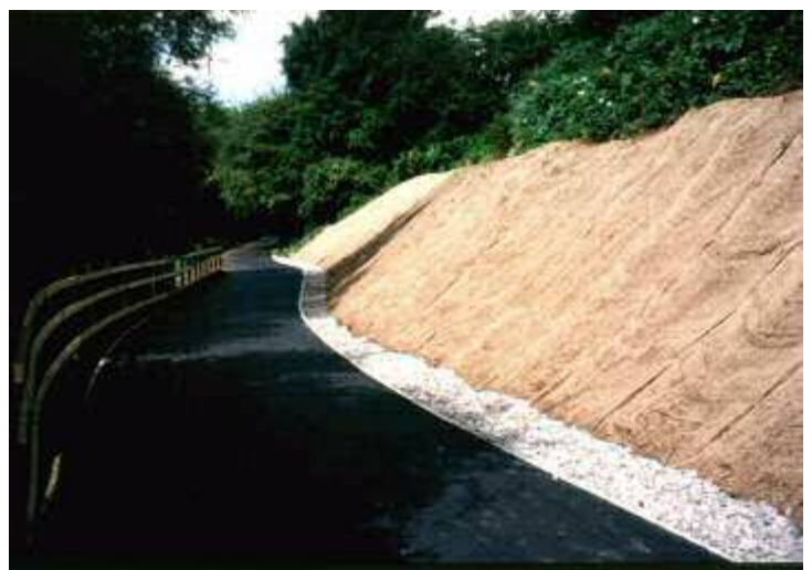
The completed cycle route with geogrids and top soil in fully stabilised embankment.
