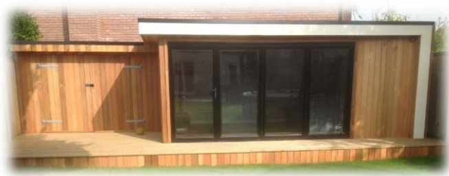
Pictured: Wilmslow - 6 x 4m room with 4 x 1.5m shed on Anchor Post foundations
