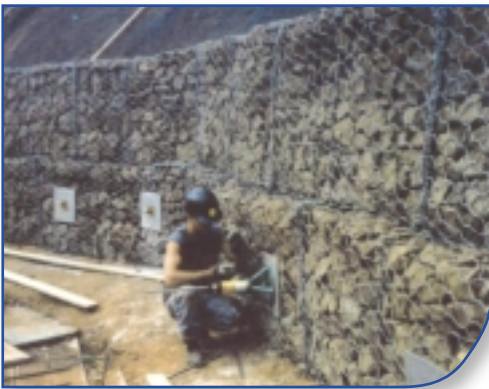
Gabion Baskets Nelson Close, Exeter
