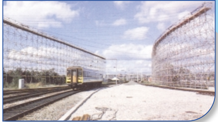
Scaffolding Power lines crossing railway tracks
