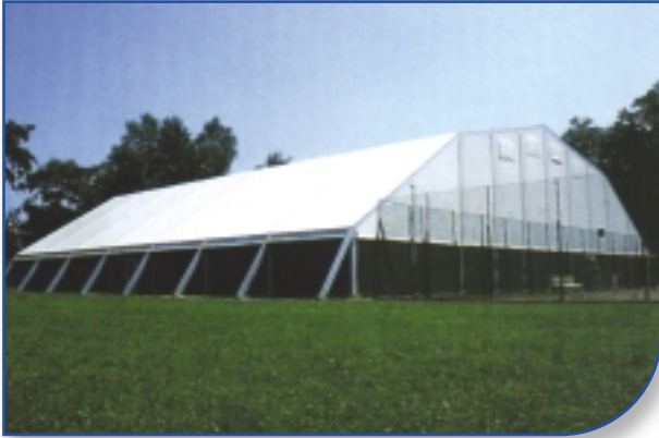
Tennis Court Covers Garrison Tennis Club, Strasbourg, France
