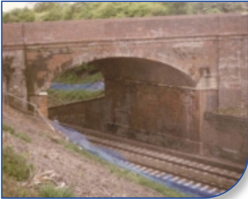
Bridge Abutments London to Brighton Mainline
