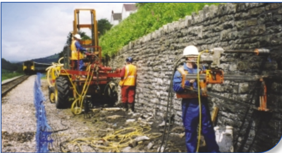
Retaining Walls Merthyr Vale
