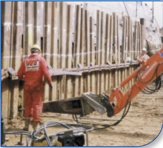
Sheet Piling Docklands Light Railway
