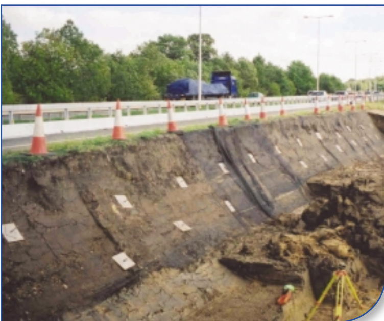
Embankment Stabilisation The A2 at Boughton
