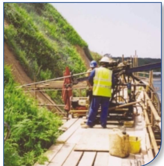
Cliff Stabilisation Nefyn, Gwynedd, North Wales
