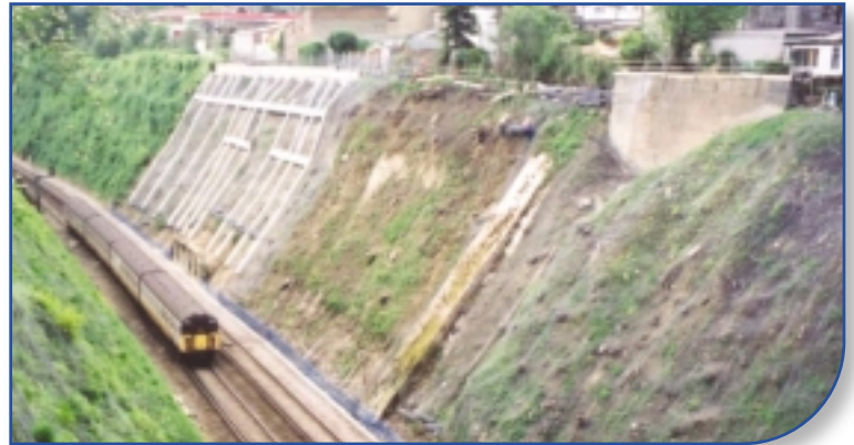
Geotextiles Merstham Cutting, Croydon
