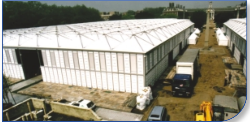
Temporary Relocatable Structures Chelsea Flower Show
